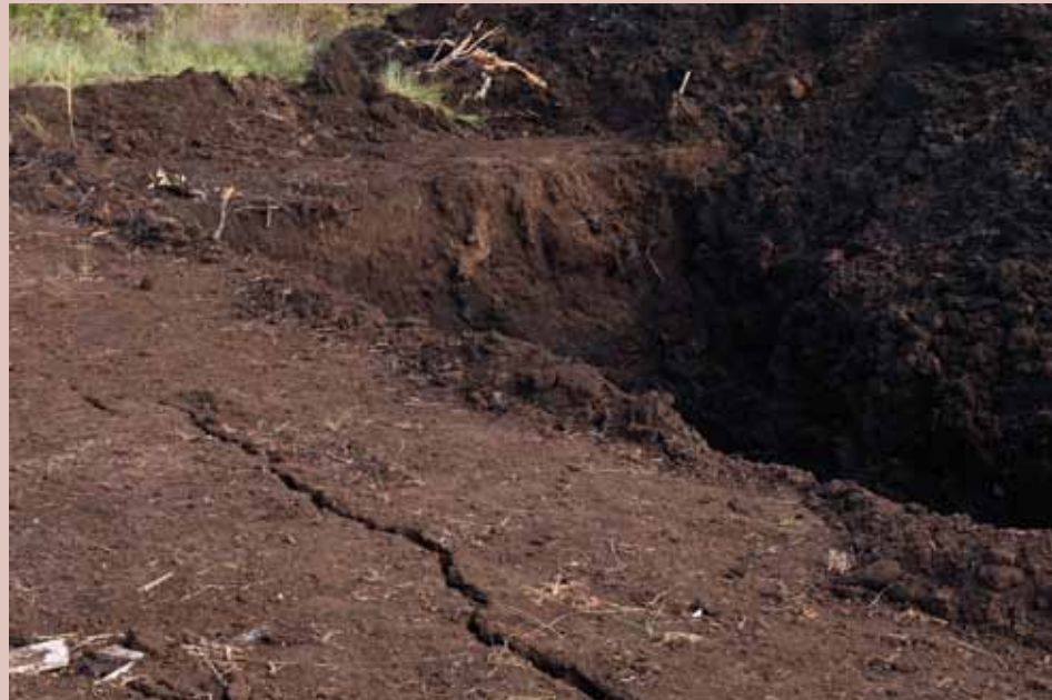
Collapsing side walls were a common feature at this location
