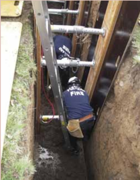
Trench rescue training conducted by Portland Fire and Rescue
