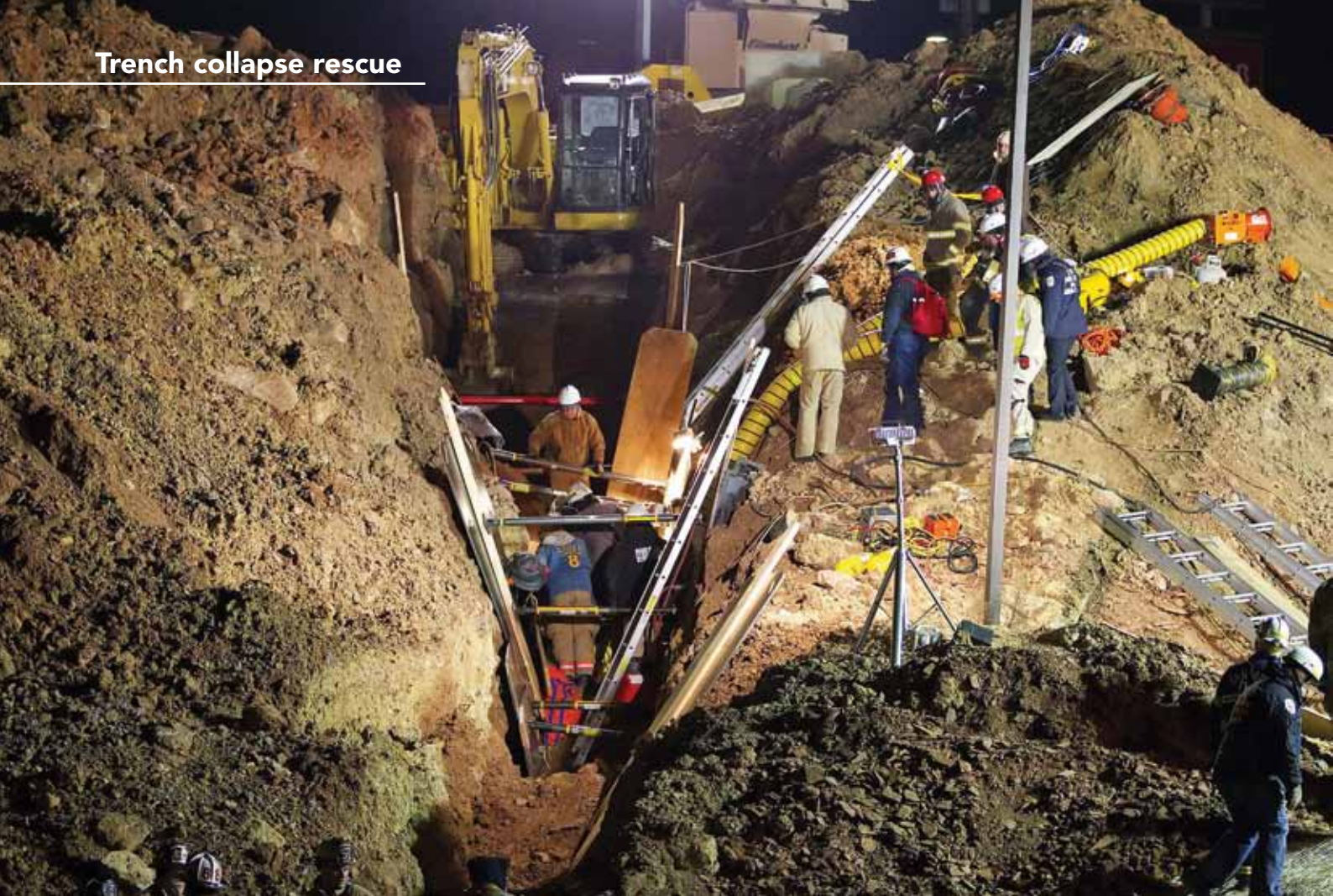
Trench ventilation should be on-going throughout the trench rescue operation
